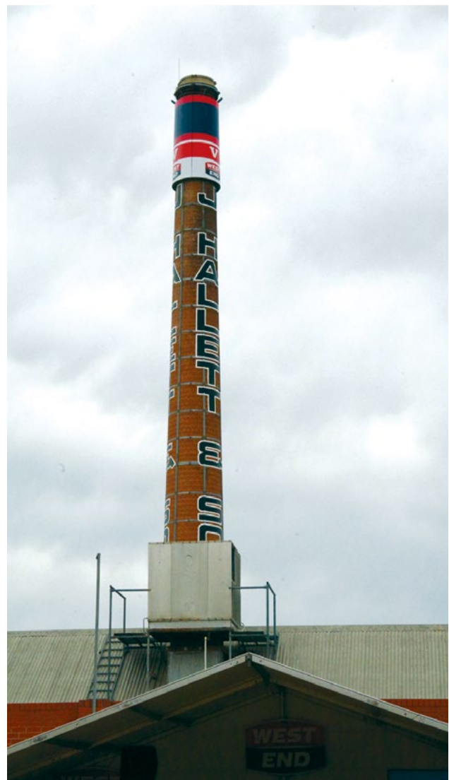
Norwood colors proudly on top of the Brickworks chimney Photo - John Emery.
